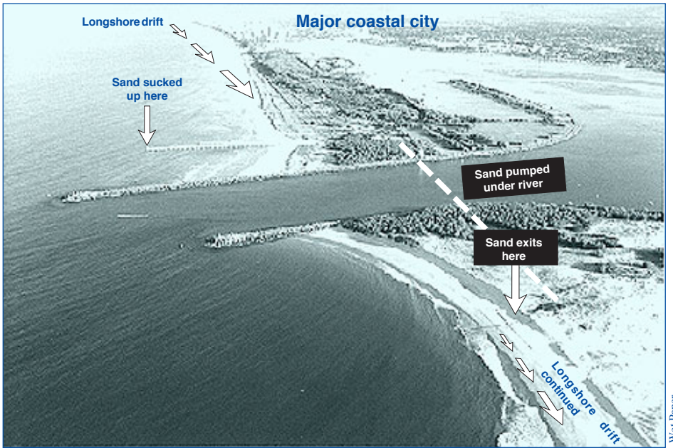
Figure 21.1 Longshore drift and the Nerang River entrance
